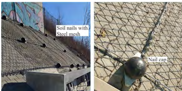
Figure 13. Soil nail with steel mesh.
